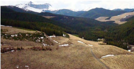
Example of reclaimed waste dump with soil cap, hummocky landform design and vegetation.
