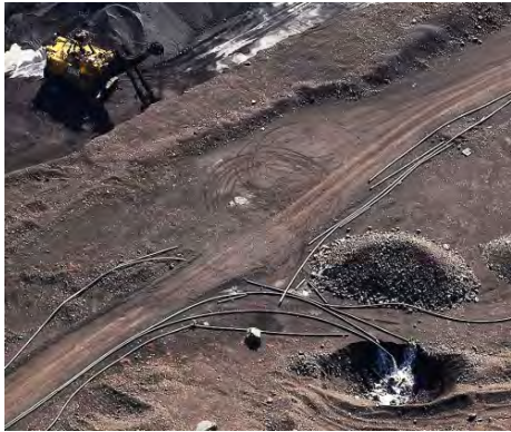
Diverting water into a rock drain.
