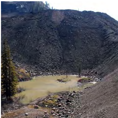
Ponding of creek upstream of a rock drain.
