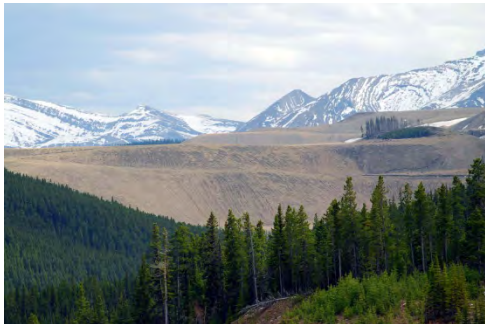
Two examples of legacy waste rock dumps.
