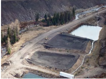
Construction of pilot passive treatment system.
