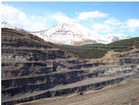
Active Pit Where Backfilling is Occurring
