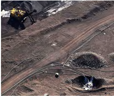
Diverting water into a rock drain.
