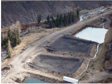
Construction of pilot passive treatment system.
